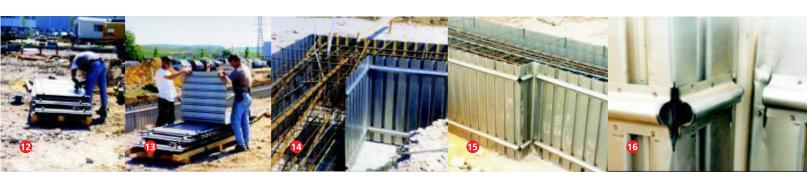
Formed parts, such as interior or exterior edges, are created with a right angle grinder through cuts into the cross-sections and bending them to the desired shape. See pictures from 😰 to 🚯
