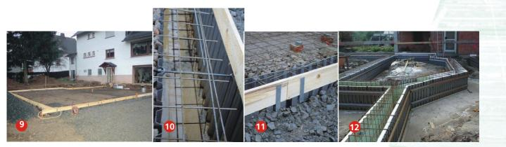
The base plate and the foundations can be shuttered simultaneously (please refer to the FS 2001 light specifications on this). Another client variation for base plates is shown in photos 9 to 11.
