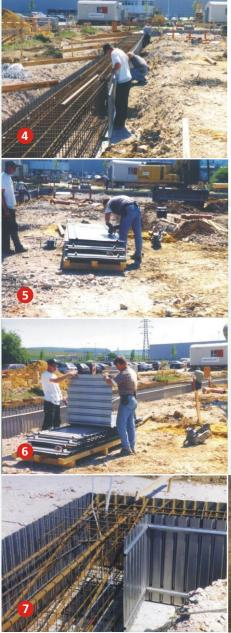
The 3.1 meter lightweight foundation wall shutter ing element adheres to its shape thanks to 27 vertical trapezoidal profiles.
