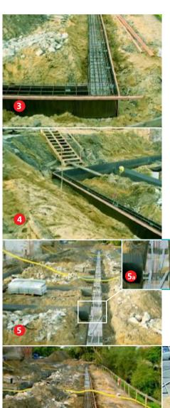
MSL - girder casing system Type FS-U-Shaped
