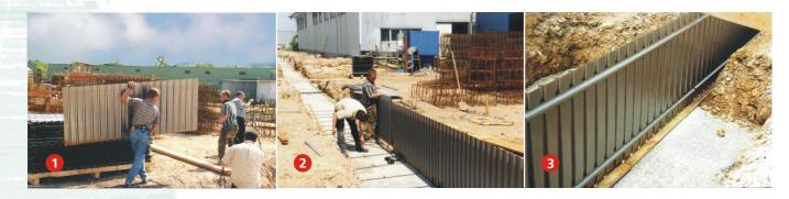
MSL FS 2001 foundation shuttering consists of only two components. 1) Foundation wall shuttering element 2) Insertible connector
